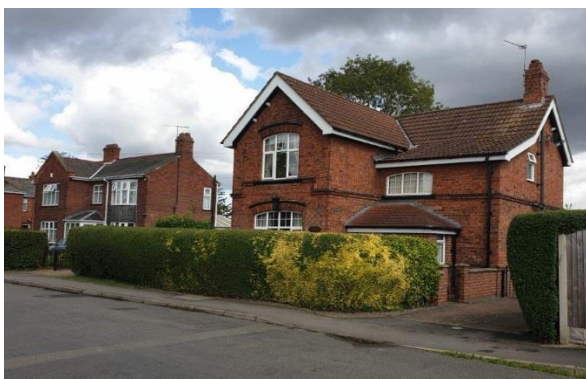
7 – Traditional interwar houses (originally local authority) on Walkerith Road (Nos. 34-54). Three blocks of 4 houses each with traditional construction, brick, render and small element
