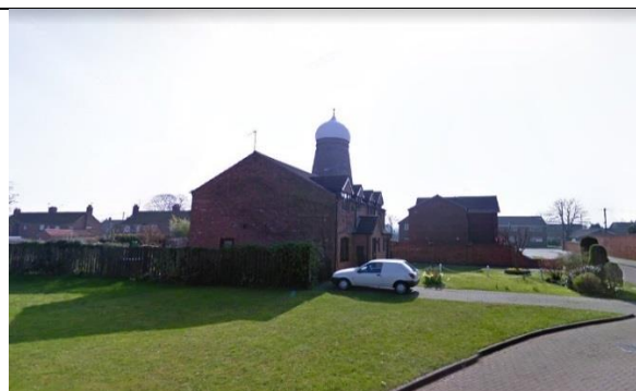
View of Mill from Granary Close
