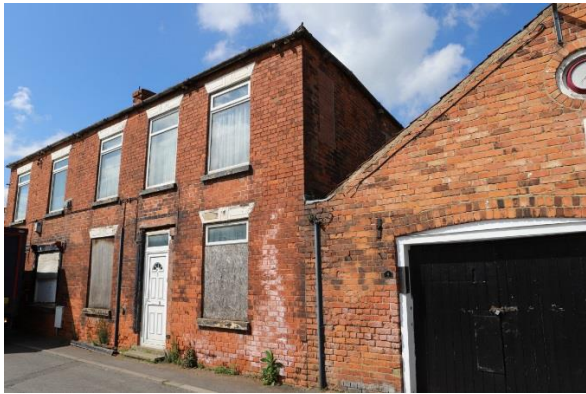
4 - St Oggs. Late C19 villa (now nursing home) original windows, brick details & ornate facias.
